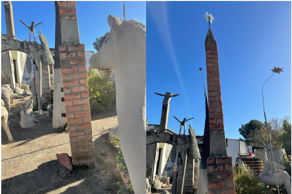
The Leaning Tower before the repair
